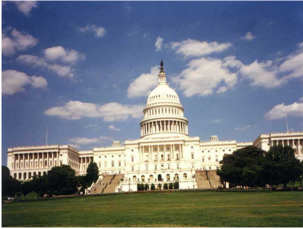
The Capitol Building
